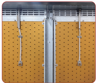
全程氧气浓度巡检取样口 Sampling port for whole-process oxygen concentration inspection
